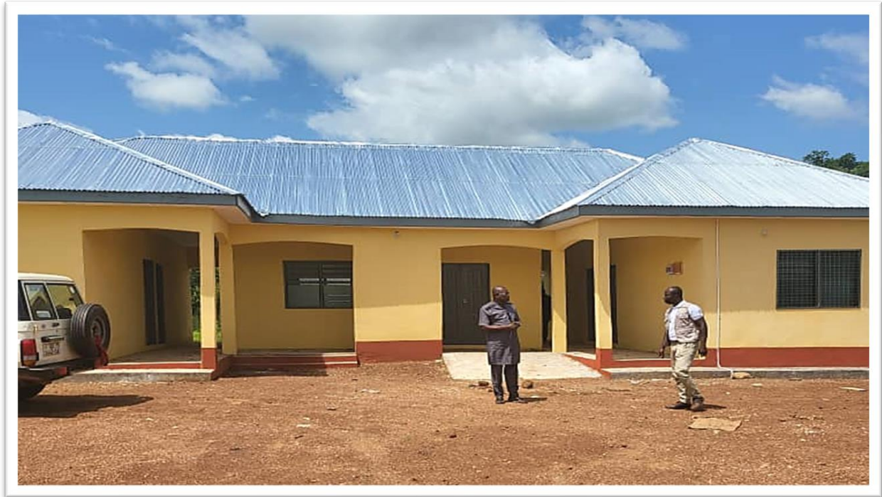
CHPs Compound at Jakpumba
