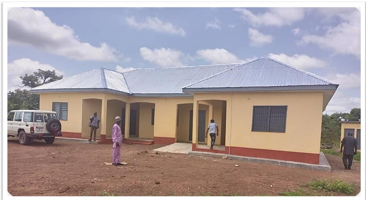
Constructed 1 No. CHPs Compound at Kanjonayili
